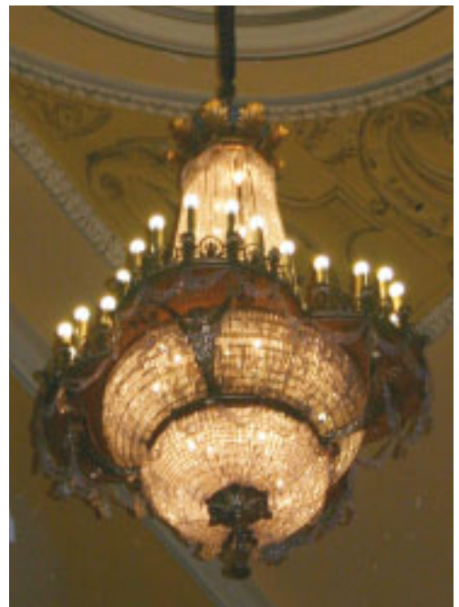
(Top) Efficient lamps can often be retrofit inexpensively without changing the existing light fixtures.
