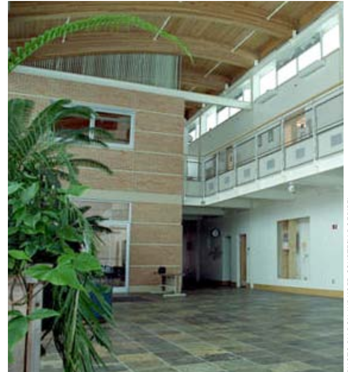
The atrium at Oberlin College's Adam Joseph Lewis Center for Environmental Studies uses daylighting to significantly reduce the electrical loads of the building.
