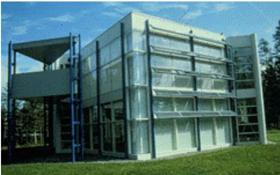
PV shade screens (Finland)
