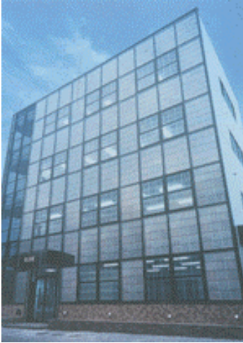
PV facade integrated with clear glass (Sanyo Building, Japan)
