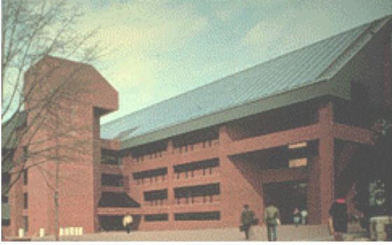
Georgetown University's 300 kW PV roof in Washington D.C.
