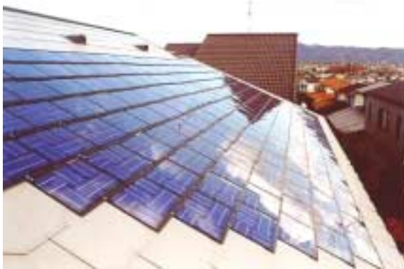
PV slates were developed in Europe, where slate rooftops are common. PV slates can also replace shingles (Atlantis Solar Systems)
