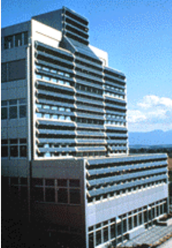
PV shade screens (Switzerland)
