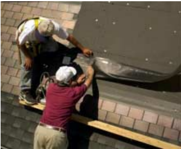
Photo 1 Installing UniSolar PV Shingles
