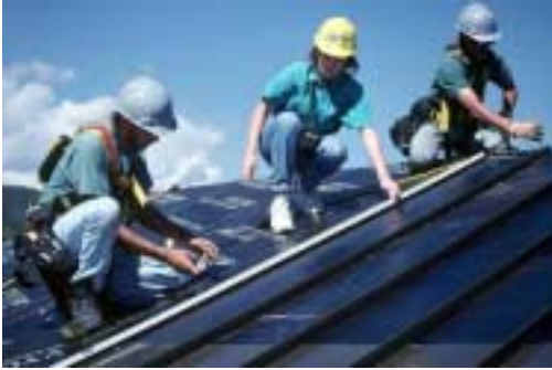
Photo 3 Installing UniSolar standing seam PV roofing
