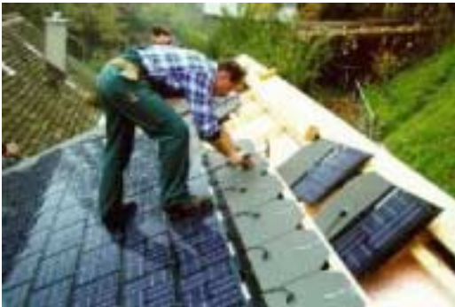
Photo 4 Installing Atlantis Energy's SunSlates
