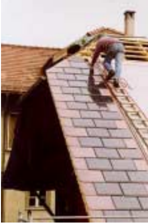
Photo 2 Installing Atlantis Energy's PV Shingles
